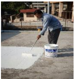
Roof surfaces of existing buildings
