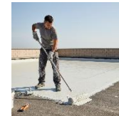
Acrylic coatings on roof surfaces
