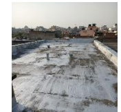
Over flat roof surfaces
